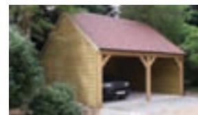
OAK FRONTED CARRIAGE HOUSES
